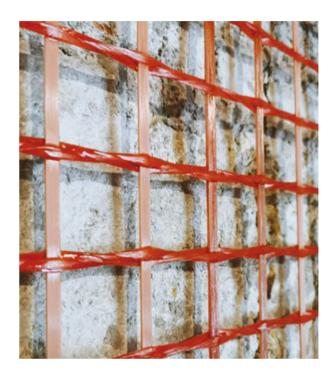
With the new CRM reinforced plaster systems of the Olympus STONE line it is possible to carry out interventions that are compatible with the masonry and do not present particular criticalities. Per definition a CRM system has a thickness between 30 and 50 mm net of the possible leveling of the support.
