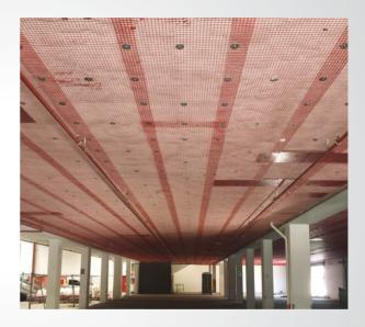
to the load-bearing capacity, can cause losses in economic terms and in human lives. These elements have been the source of collapses that have led to the uninhabitable of buildings and to losses and risks to human life. The absence of oxidation phenomena also ensures high durability over time of these systems, eliminating of these systems, eliminating the typical criticalities of the traditional interventions.
