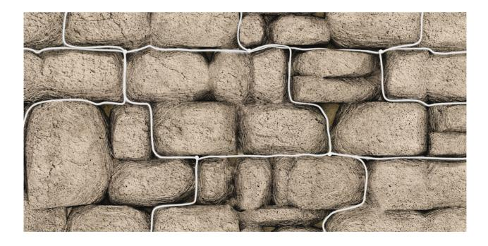
This technique can be used both to reinforce the single masonry panel and to reinforce an internal structure, also creating an effective connection between transverse walls thanks to the continuity of the steel cables that go to reinforce the mortar joints.
